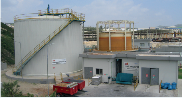
Pepsi Co Gıda - Frito Lay Tarsus Solid Waste Treatment Plant 3.000 m 3 Anaerobic digester (40.000 ton/year; 500 kWe), 2010
