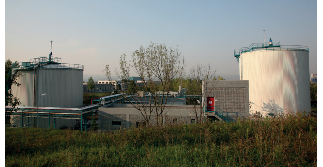
Pepsi Co - Frito Lay İzmit Potato and Corn Chips Factory - Solid Waste Treatment Plant with 4.000 m 3 Anaerobic digester and (50.000 tons / year; 330 kWe) capacity is the first application of Arbiogaz for solid waste treatment plant, 2008
