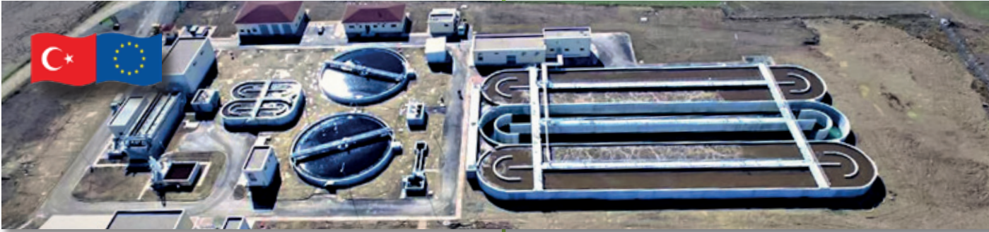
Akşehir Wastewater Treatment Plant and Wastewater Collectors 15.000 m 3 / day
